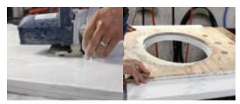
Rough out the sink with a blade and clamp template in place
