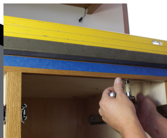
Adjust Shims From Below
