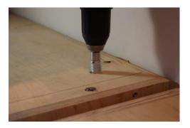
3. After the counter is in place, adjust the level from the underside using the custom driver and 3/8" socket & ratchet combination.
