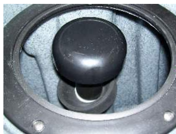
Float Shutoff Assembly
