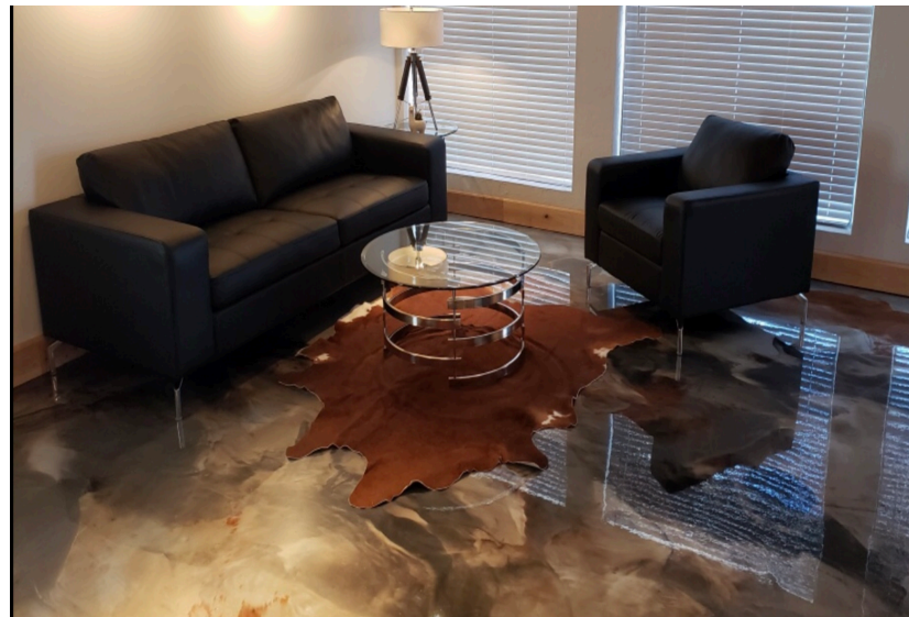
Epoxy LV applied at 55 sq. ft per gal or 25-30 mils
